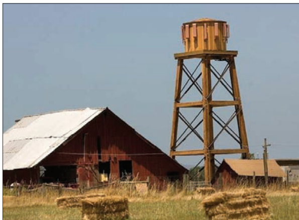
Rusty rooftops and fences can be prime sources of PIM
