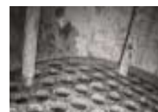
Corrosion of heat exchanger end plate
