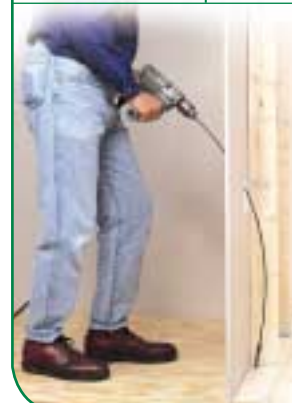
Flexible steel drill bits are perfect for installing wire or cable inside existing walls.
