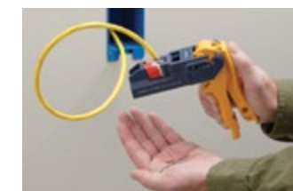
6. Wires will be seated and cut for a solid termination.
