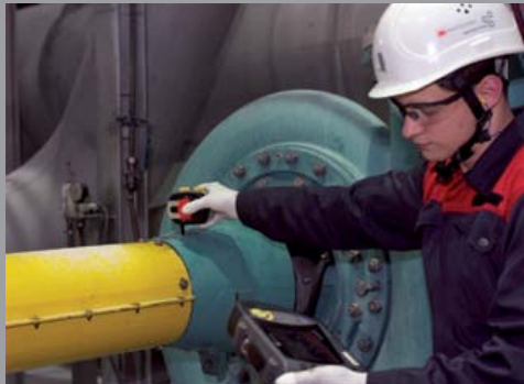
Vibration measurement The good alignment should be confirmed by reduced vibration values.
